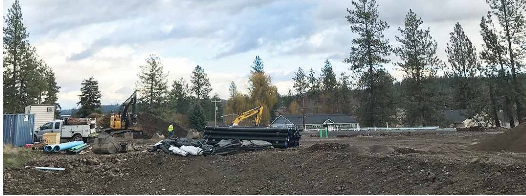
Construction is underway for new apartments and a new ECEAP center.
