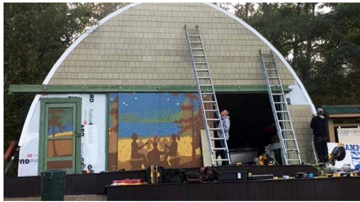
In 2020, staff did renovations to Camp Cross facilities.
