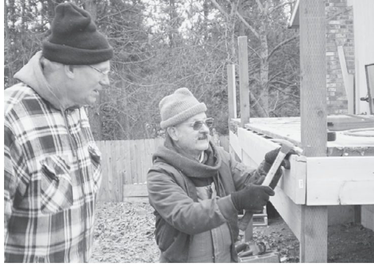
Bob Granger and Tom Collier work on a porch repair.
