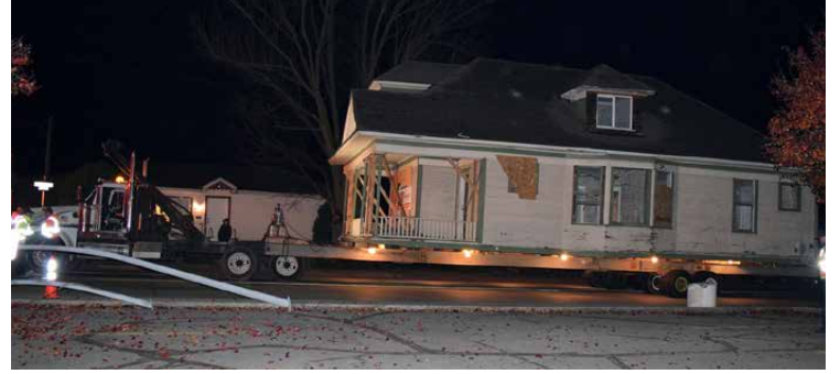
One house is moved in West Central Spokane. Photos courtesy of Deb Conklin
