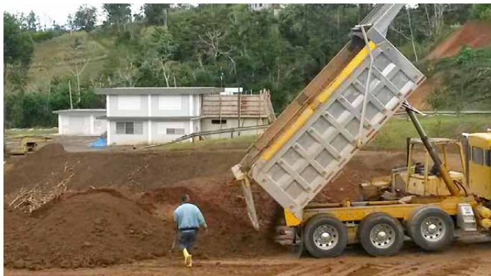
Equipment cleans up landslide after a recent rain. Dorm where team is staying is in the background.
