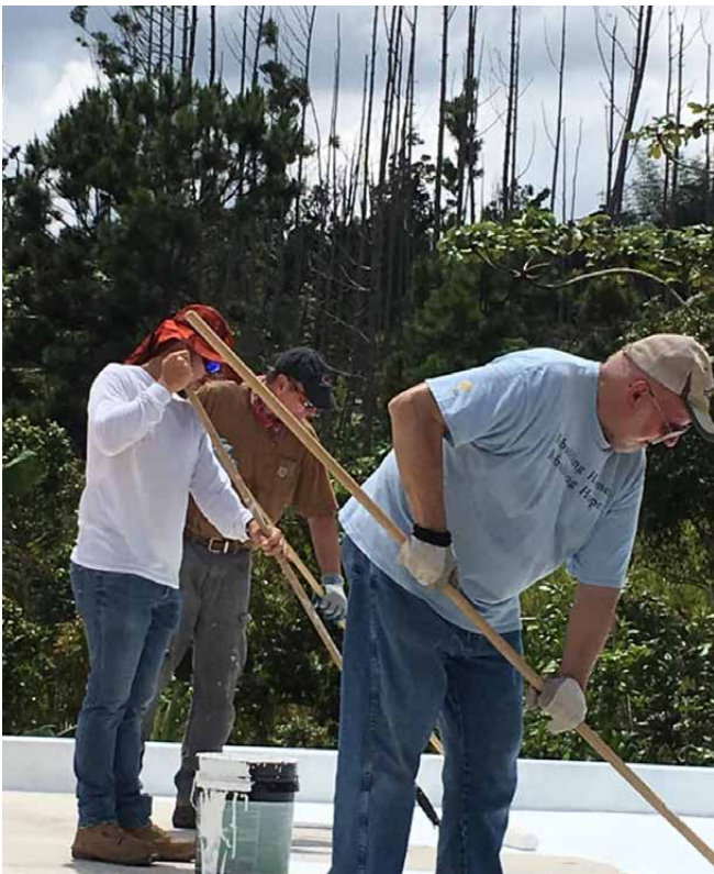
Behind a team sealing a roof in Puerto Rico are pine trees that were damaged in Hurricanes Maria and Irma.
