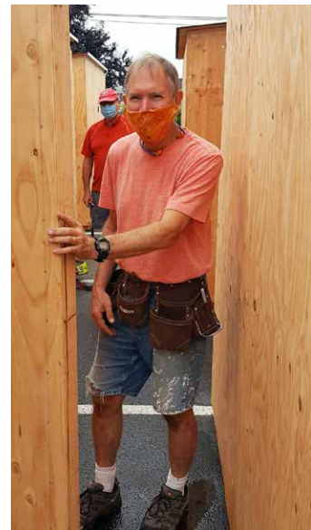
Jeff Loyer at work on building.
