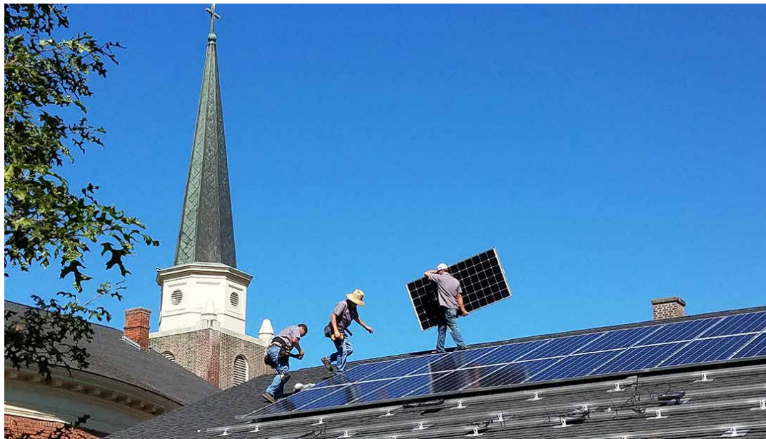
Crew mounts solar panels on the roof of First Congregational UCC in Walla Walla.
