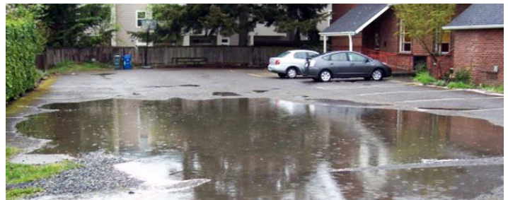
Broadview UCC's parking lot becomes a 18-inch lake in Seattle's rainy season.
