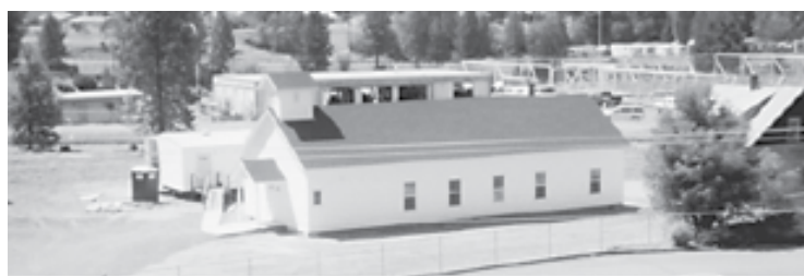
Progress is being made on the church building and siding has been added to adjacent building.
