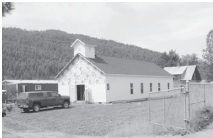
Siding installation on the new church.
