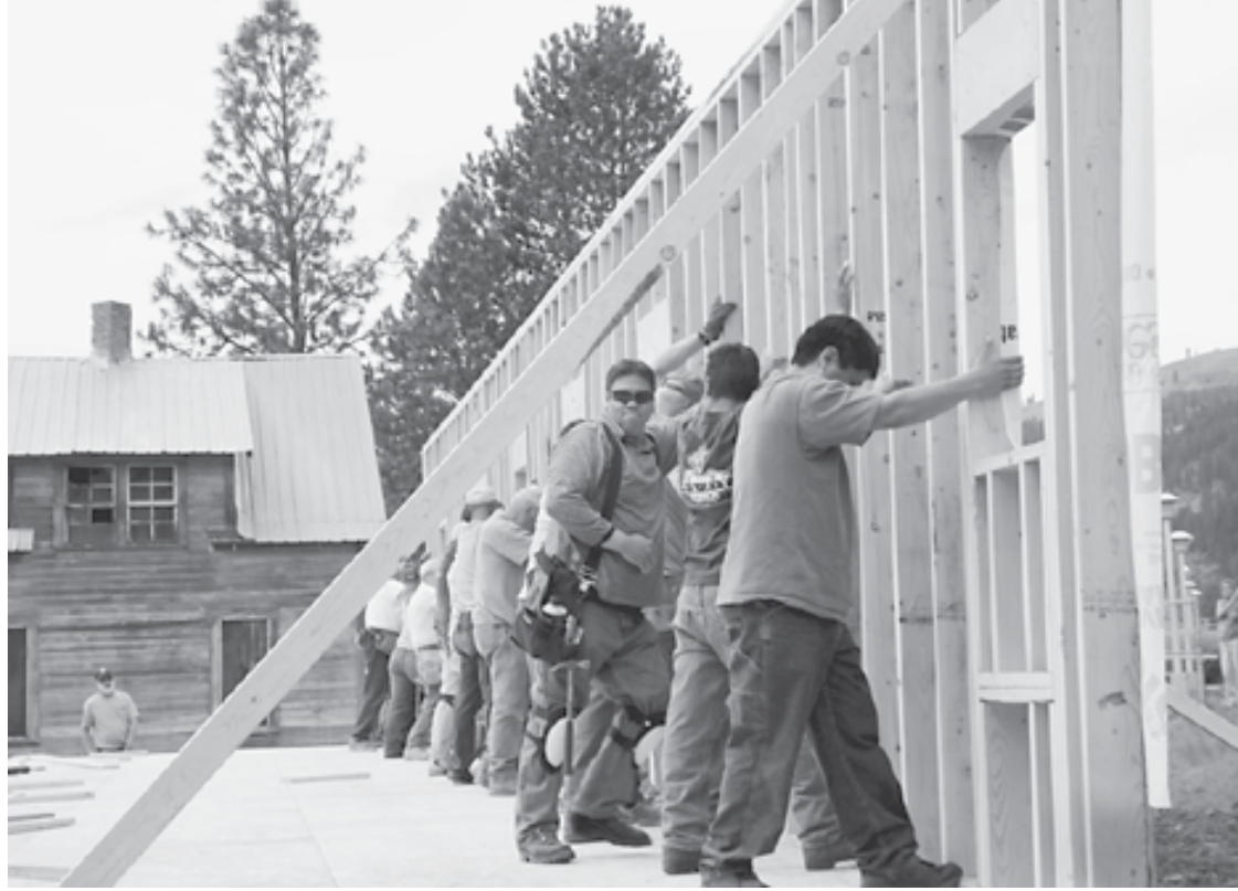
Members, community and neighbors helped raise the walls in March.
